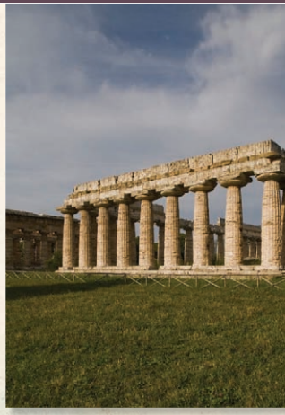
Temple of Hera, Paestum. Ca. 560–550 BCE. Limestone. Archaic temples set up used by the Greeks. The buildings were aligned east-west, with the entrance to the altar stood before the entrance, and people gathered around it to stage a sacrifice enclosed space inside the temple’s colonnade was off-limits except to the priests
