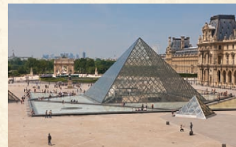
Louvre Pyramid, Paris. 115 on each side, 70 high. This glass and steel pyramid designed by I. M. Pei (1917–) opened in 1989 as the main entrance to the Louvre Museum. Pei's pyramid was in part a homage to the precise geometric designs of the great French landscape architect, André Le Nôtre. And, in part, the pyramid's geometric planes echoed the articulated planes of the Louvre's roof and surrounding buildings.
